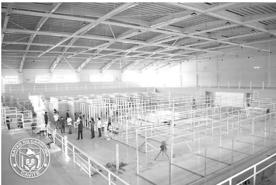
Carmona Mayor Roy Loyola visits CarSiGMA Gymnasium for inspection. Municipal Mayor Roy Loyola conducted an inspection at the CarSiGMA Gymnasium on August 18, 2020 where an additional isolation facility is being placed.
