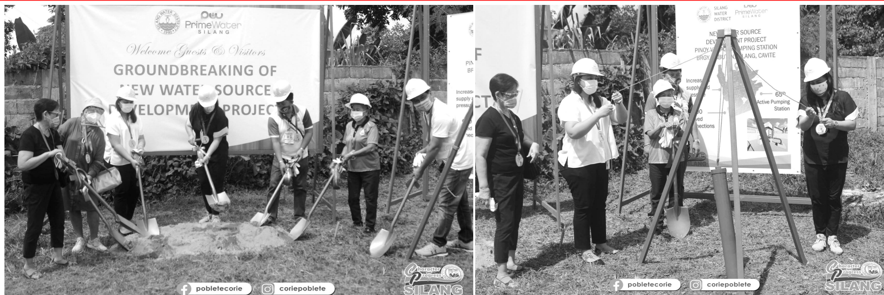
Silang Mayor Corie Poblete Ground Breaking Ceremony of Proposed Pumping Stations at Pinoy Village, Brgy Sabutan and Sitio Banaba, Brgy San Miguel 2, July 8.
