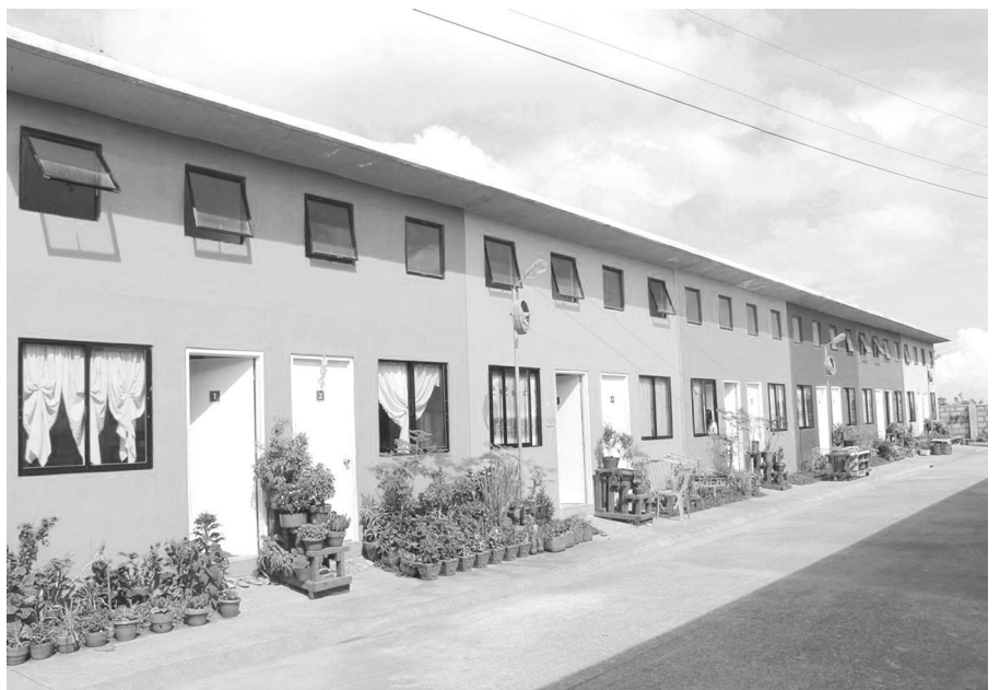
The SM Cares Village in Bogo City, the first of the four Villages constructed by the SM Group, is located in a one-hectare lot in Barangay Polambato, Bogo
